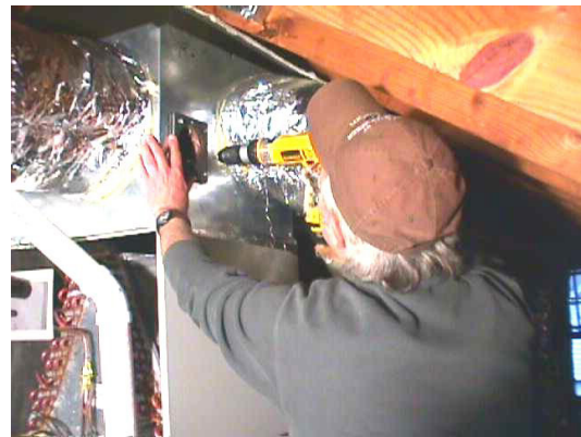
2. Install Mounting Plate
