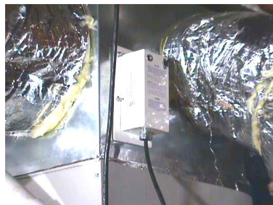
4. Tighten 4 Wing Nuts supply power from wire grounded 120V circuit, ensure LED is on
