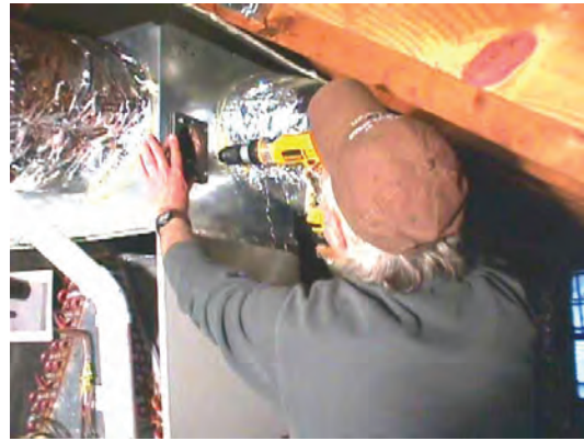
2. Install Mounting Plate
